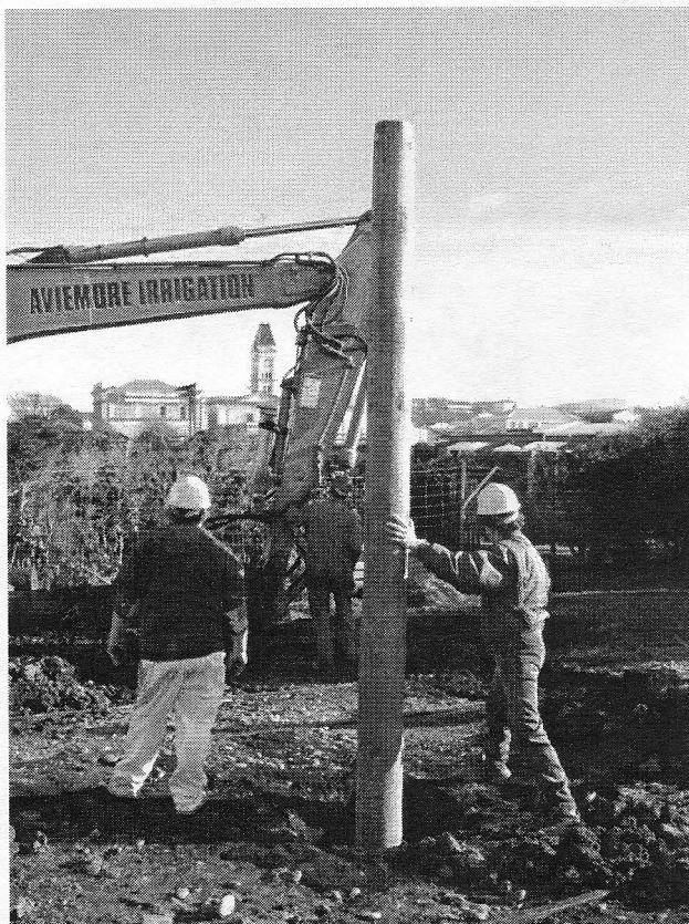
Piles being driven in for the shed extension
