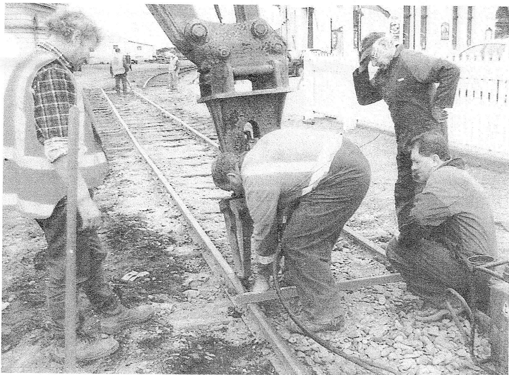
Contractors, watched by Oamaru Steam Society members Bruce Bouteray and Rick Ramsay, check the gauge of the track alongside Harbourside Station. The realigned route can be seen cutting straight across the Humber Street crossing at the top of the picture, with the end of the curve of the former route on the right.
